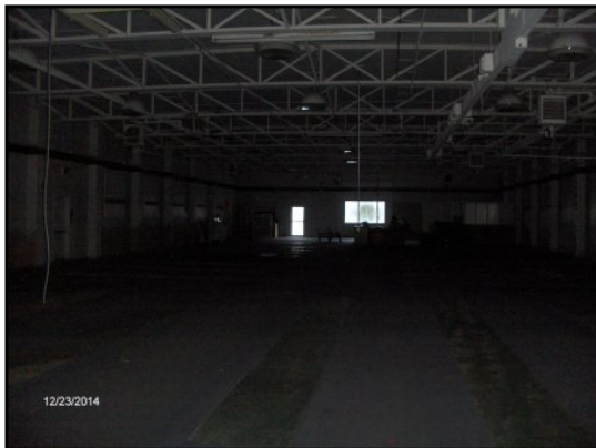
Open area of the northwest portion of the Site building.
