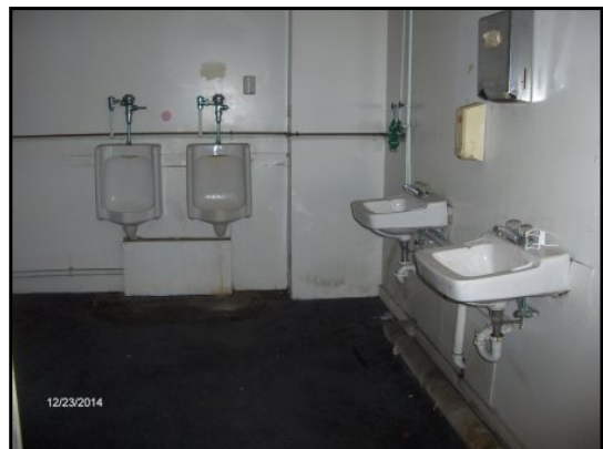
Restroom in the central portion of the Site building.
