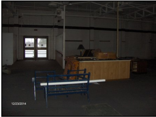
Miscellaneous storage in the northwest portion of the Site building.
