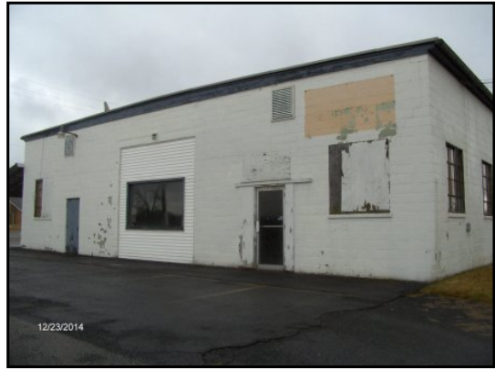
Northwest side of the Site building.
