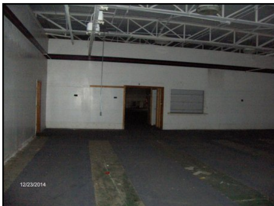
Open area of the central portion of the Site building.
