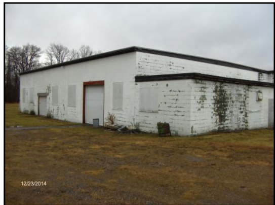
Southern portion of the Site building.
