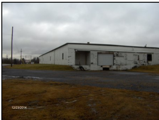
Loading dock along the southeast side of the Site building.
