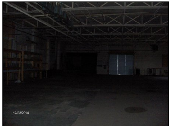
Open area of the southeast portion of the Site building.
